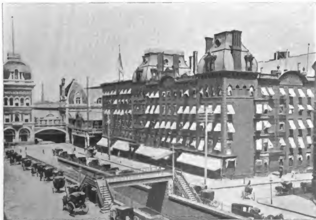
GRAND UNION HOTEL, FOURTH AVENUE, FROM 41ST STREET TO 42D STREET, OPPOSITE GRAND CENTRAL DEPOT.
